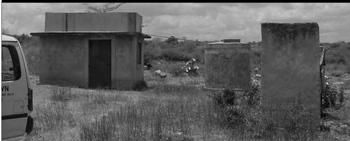
Plate 7.2: Water Storage Facility at Mtaa Dam — Kinango
