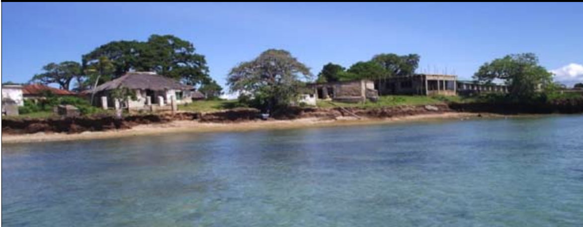
Plate 3.3: Beach Erosion at Wasini Island
